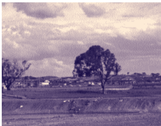
Temporary pond for trapping sediment during construction.
