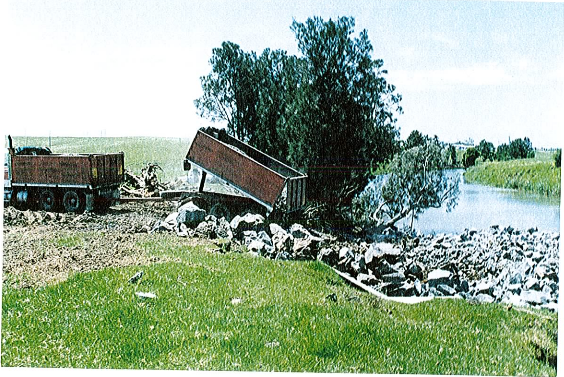
Photograph 1. Dumping of rock on site during construction of a rock-ramp fishway on McDonald's Weir, Macquarie Rivulet in January 1993.
