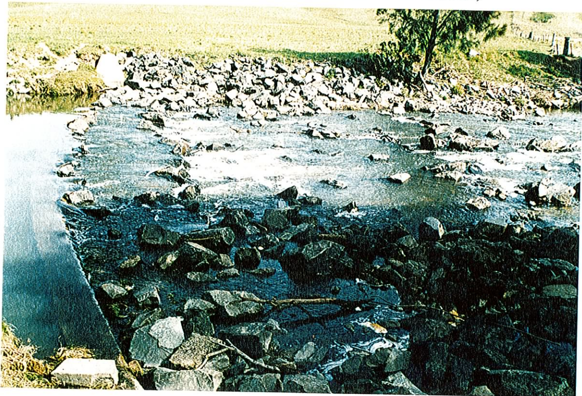
Photograph 4. After modifications to the McDonald's Weir Rock-ramp Fishway. (Note the movement of the transverse ridge rocks in the middle of the structure)
