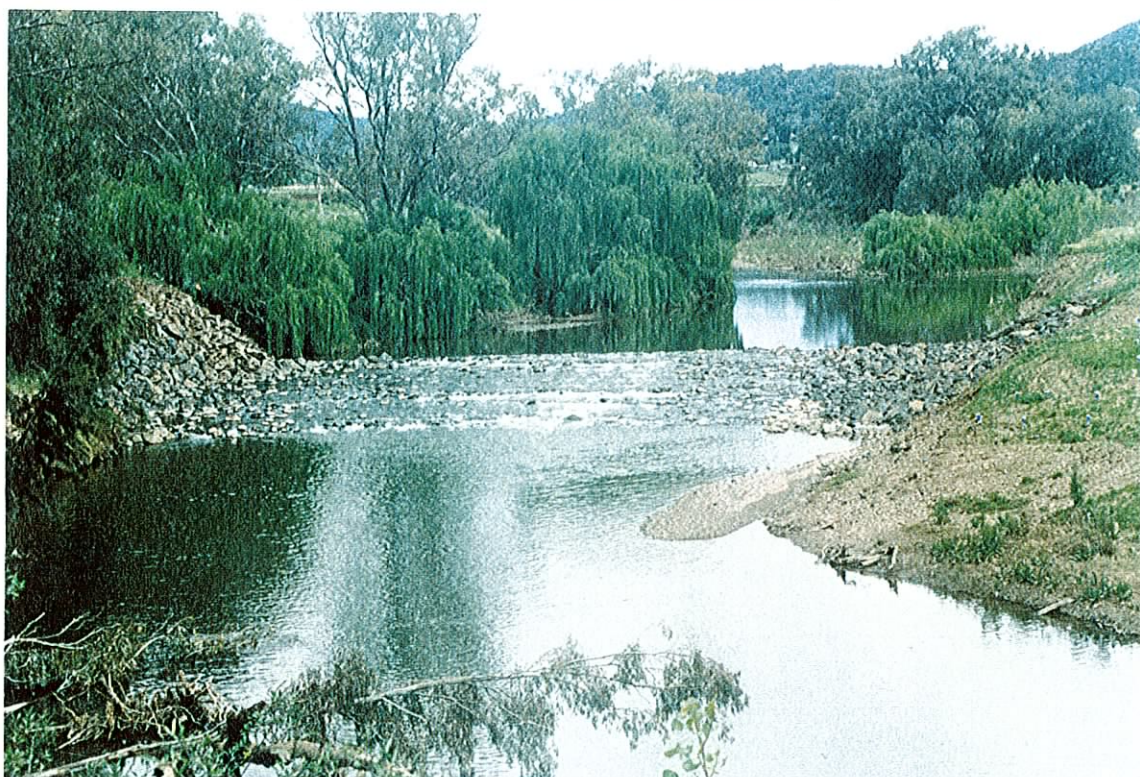
Photograph 8. After construction of the erosion control weir on the Bell River. (Note the rock-ramp fishway was formed in the centre of the structure)
