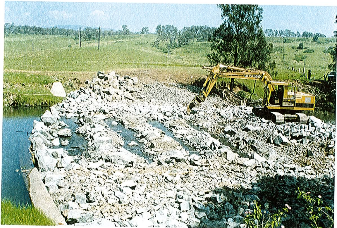
Photograph 2. Shaping transverse rock ridges during construction of a rock-ramp fishway on McDonald's Weir, Macquarie Rivulet.
