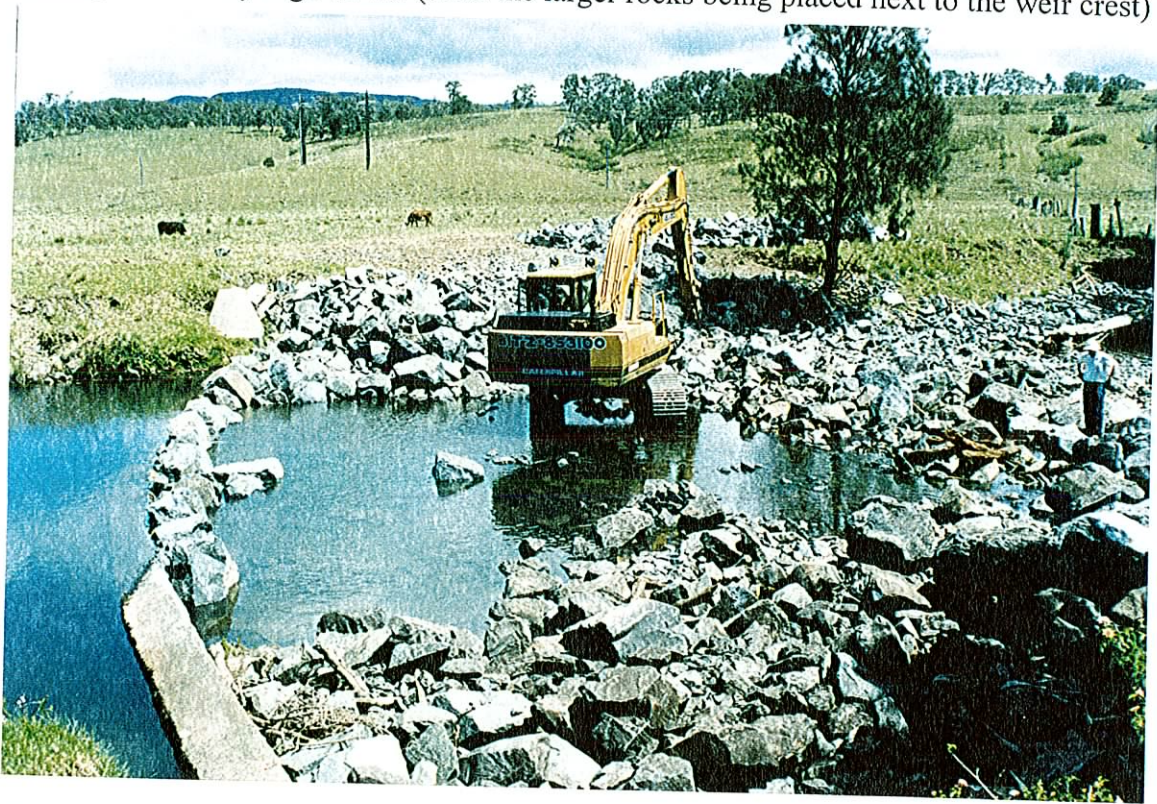
Photograph 4. After modifications to the McDonald's Weir Rock-ramp Fishway. (Note the movement of the transverse ridge rocks in the middle of the structure)
