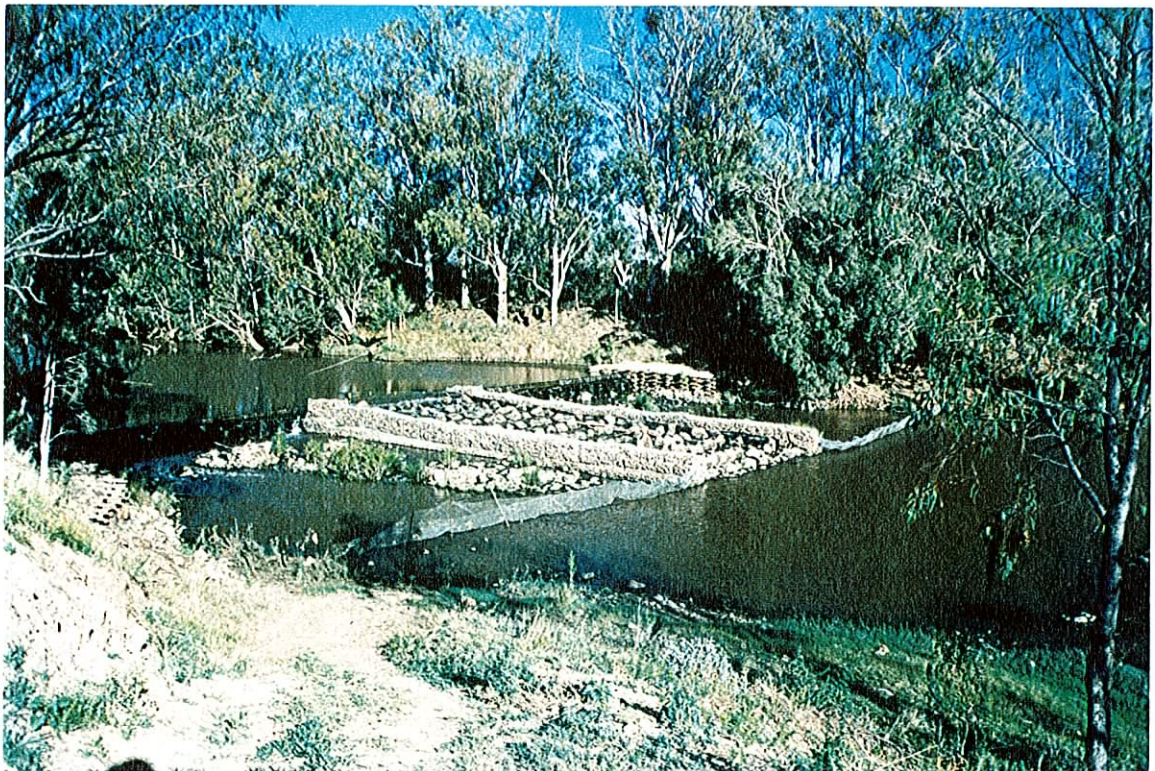
Photograph 12. Goondiwindi Weir and Fishway during sampling on 7 November 1995 with flows less than 300 ML/day. (Note lack of flow over side crests)
