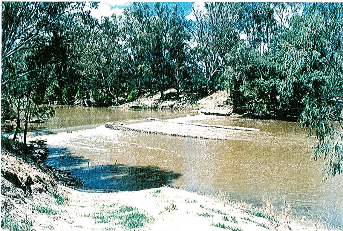
Photograph 13. Goondiwindi Weir and Fishway with 900 ML/day flow down the Macintyre River in March 1996.
