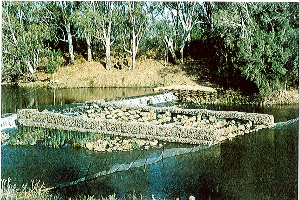
Photograph 10. The rock-ramp down the centre of the river with crests on each side of the channel raised to direct water through the fishway. (Note the guiding fence)
