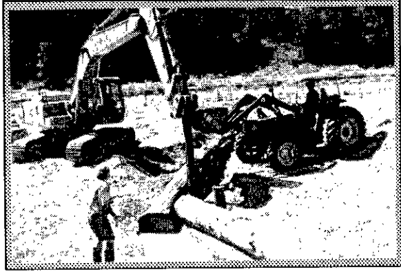
Photograph 3. NAMBUCCA RIVER, NSW. The construction of a log sill to recreate the pool/riffle sequence in a highly degraded sandbed river. NAMBUCCA River Stabilisation Task Force.
