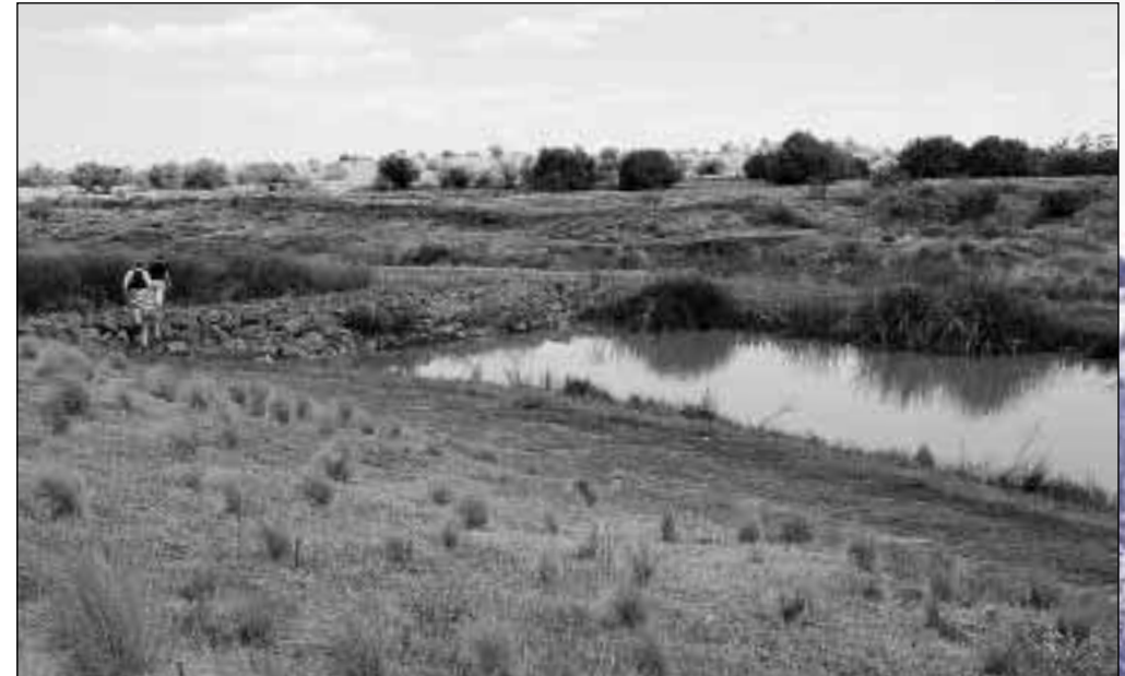
Constructed wetland inlet zone with a porous rock embankment to distribute flows evenly across the macrophyte zone. The by-pass weir is located on the far side of the open water area
