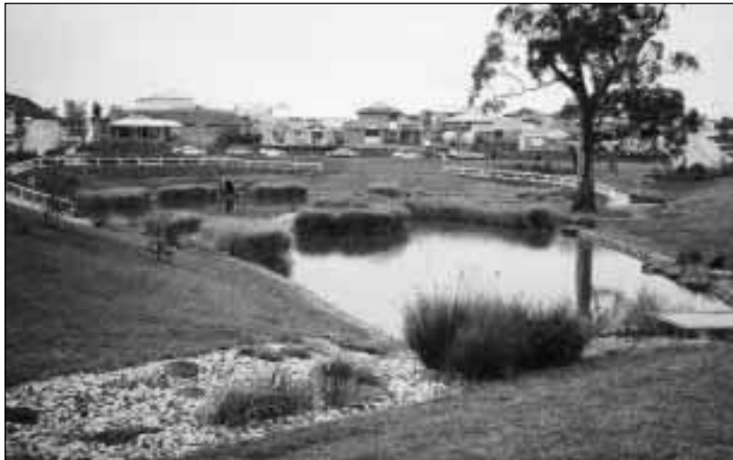
Stormwater runoff captured in a suburban pond can create an attractive water feature.
