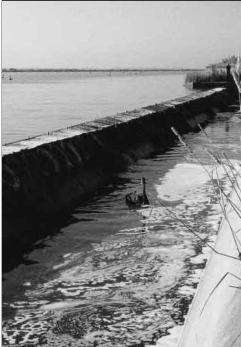
Treated wastewater discharging into Port Phillip Bay from the Western Treatment Plant
