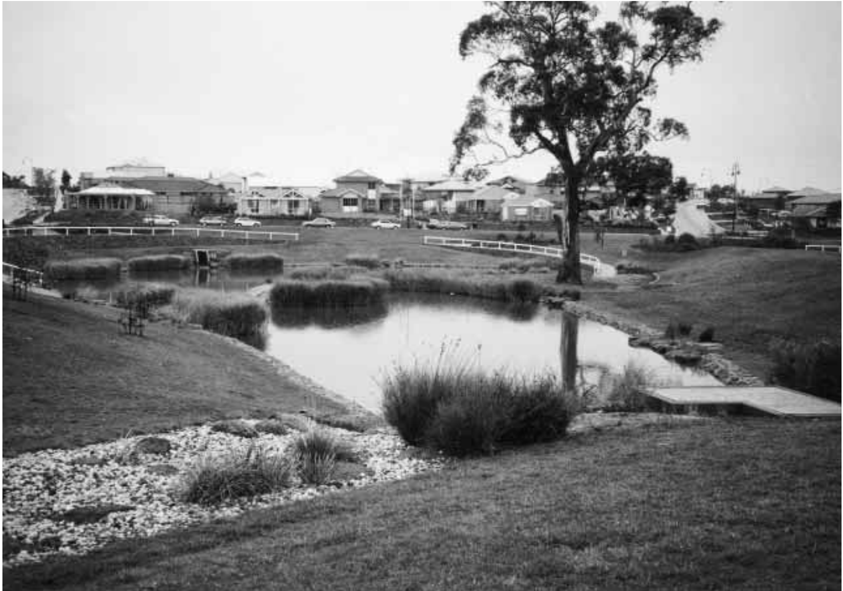
Stormwater runoff captured in a suburban pond can create an attractive water feature
