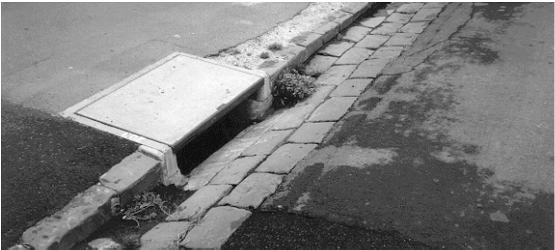
Photograph 8.2 A typical side entry pit in the experimental catchment
