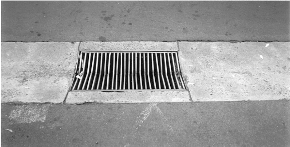
Photograph 8.1 A typical grate entrance in the experimental catchment
