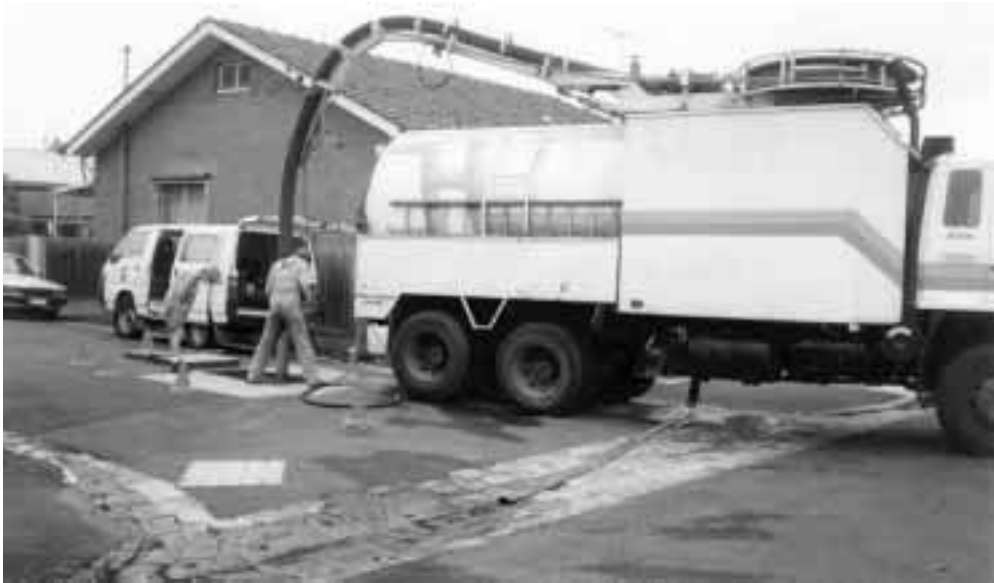
Photograph 7.1 Cleaning the CDS unit with a large vacuum device
