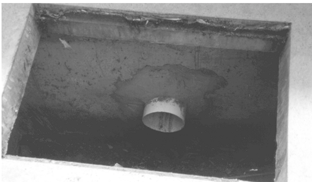
Photograph 8.4 A Coburg entrance to the drainage system that bypasses the SEPTs
