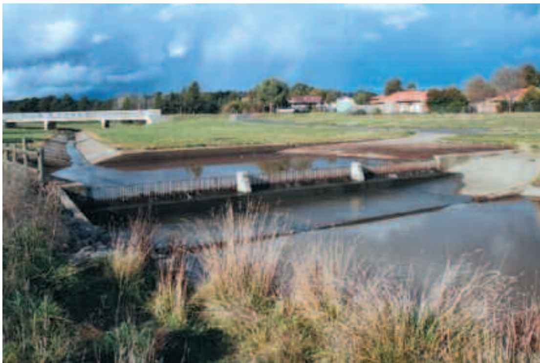
Figure 3.2 Gross Pollutant Trap Types. (Source: Ian Lawrence)
