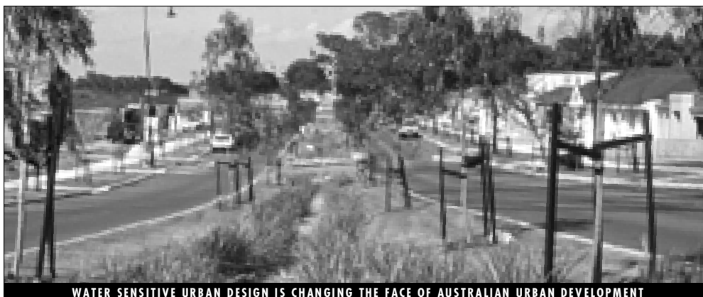
WATER SENSITIVE URBAN DESIGN IS CHANGING THE FACE OF AUSTRALIAN URBAN DEVELOPMENT
