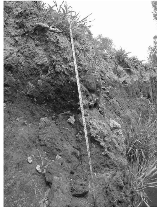
Figure 6.2: A slab failure in the foreground has removed the bank face to a depth of ~20 cm. The moss is still covering the bank in the background, despite recent inundation.
