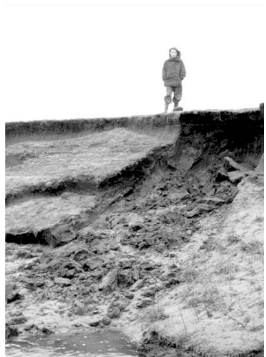
Figure 6.3: A mass failure observed at Topcliffe (2 February 1997).
