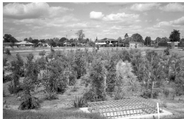
Figure 4.3 Hoyland Street Bioretention System October 2002
