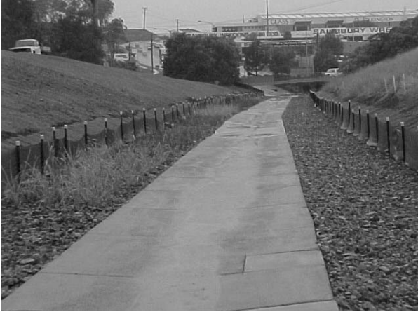
Figure 4.4 Spencer Road Bioretention System August 2002 (Photograph Colin McMurtrie)
