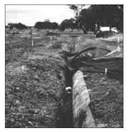
Photo 2: Construction of gravel trench
