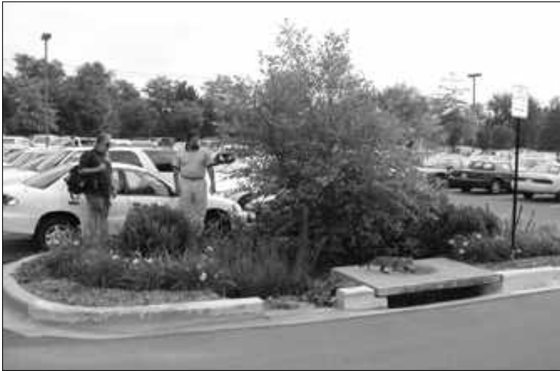
Figure 4.2 A bioretention system (rain-garden) using a combined sand and organic mulch filter media for stormwater treatment in Prince George's County.
