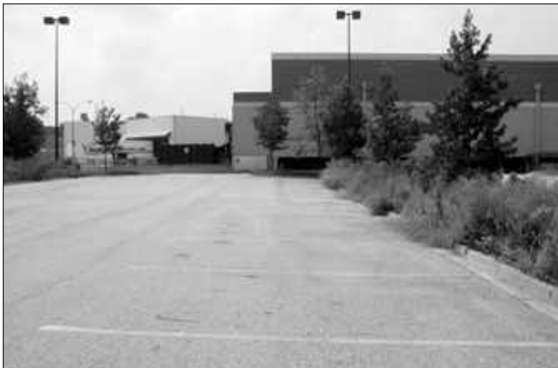
Figure 4.3 A car park design as a flood retarding basin (notice cross-fall of pavement) as well as for stormwater treatment through the bioretention median strips.
