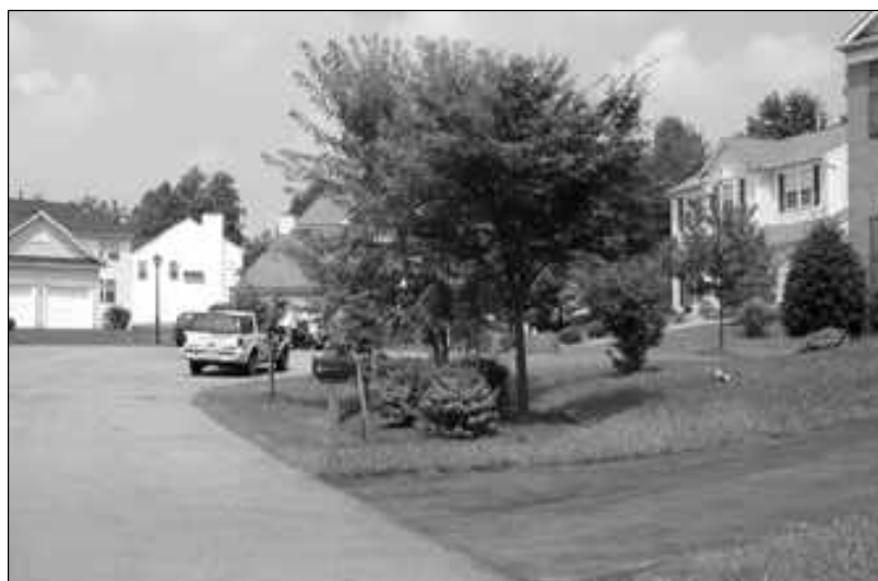
Figure 4.4 Somerset Gardens, Prince George's County, Maryland – A Low Impact Development using a combination of grass swales and rain gardens for stormwater conveyance and treatment.
