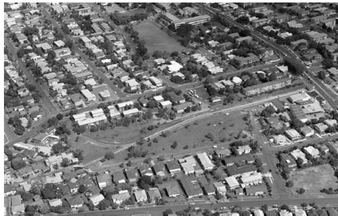
Figure 4.2 Bridgewater Creek - prior to the construction of the wetland
