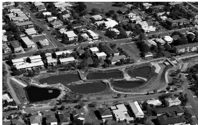
Figure 4.3 Bridgewater Creek - post-construction
