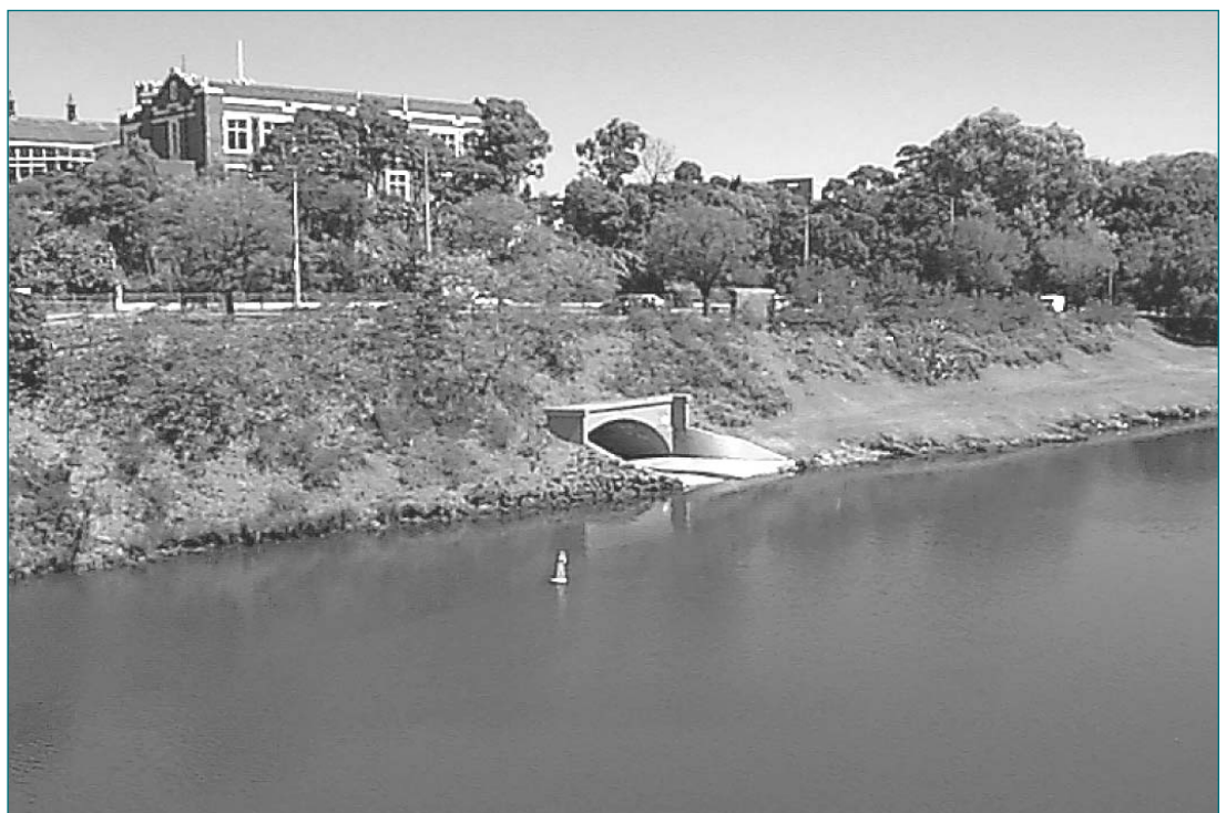
Figure 5.1, The Prahran Main Drain outlet to the estuarine reach of the Yarra River – a typical example of a pollutant source in extremely urbanised catchments
