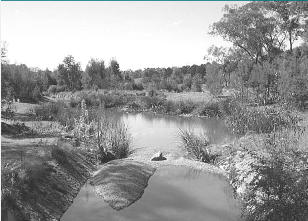
Figure 5.2, A sediment trap at the entry to the Ruffey Lake wetland. The stormwater receives treatment before flowing into Ruffey Lake in Doncaster. Below the lake, Ruffey Creek flows into the Yarra River at Templestowe.
