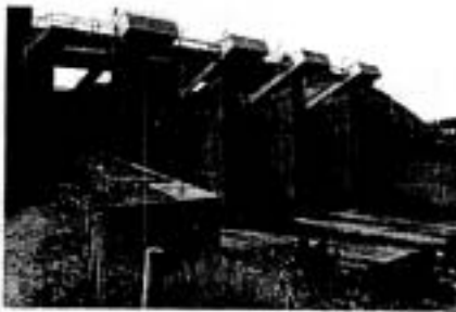
Figure 4.16c: Downstream view of the dam wall of Sno 06.
