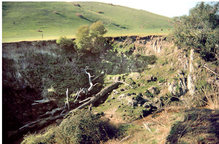
Plate 1. Extensive erosion in upper catchment of Creightons Creek in the Granite Creeks System (Photo: Sam Lake)
