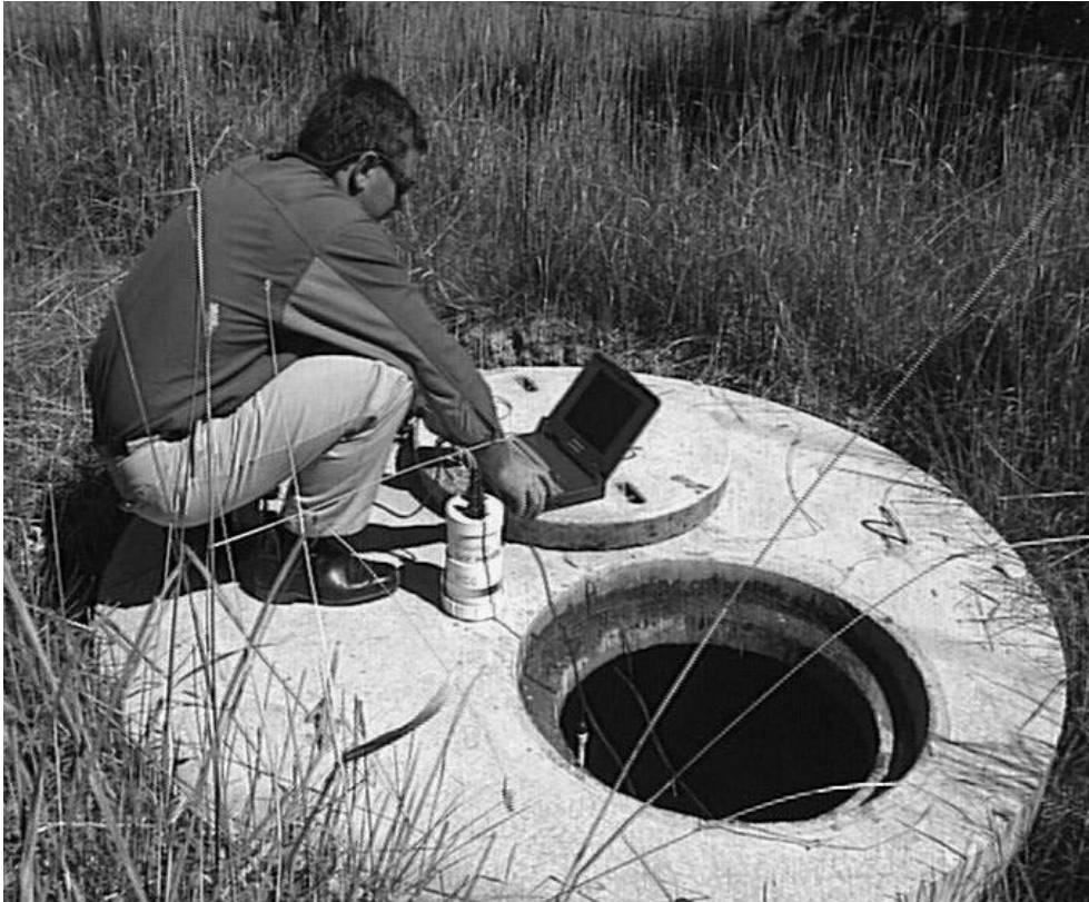
Figure 3.2: Flow logger and sewer access point
