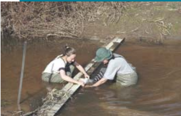
A red-gum structure installed over a sand slug. Photo: CRCFE
