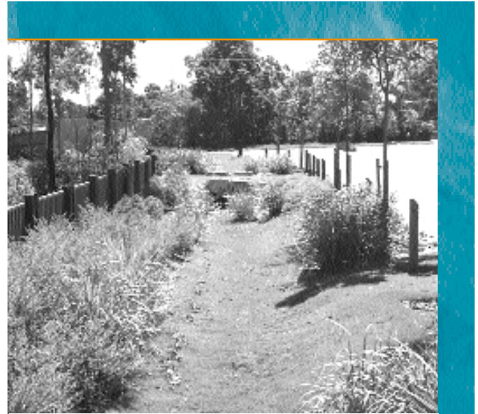
Grassed swales allow stormwater to infiltrate the soil and travel slowly to streams. Photo Tim Fletcher
