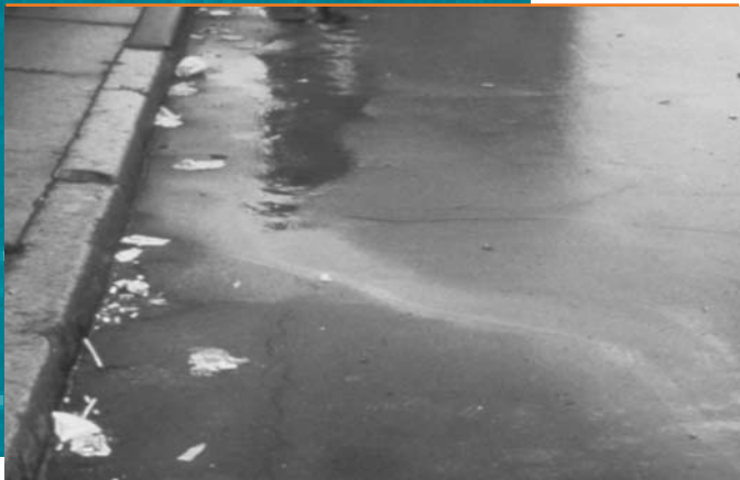
Traditionally, oily water and contaminants drain off roads and into stormwater pipes that carry them directly to urban creeks.
