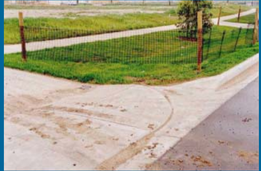
Grassed swale in street verge*
