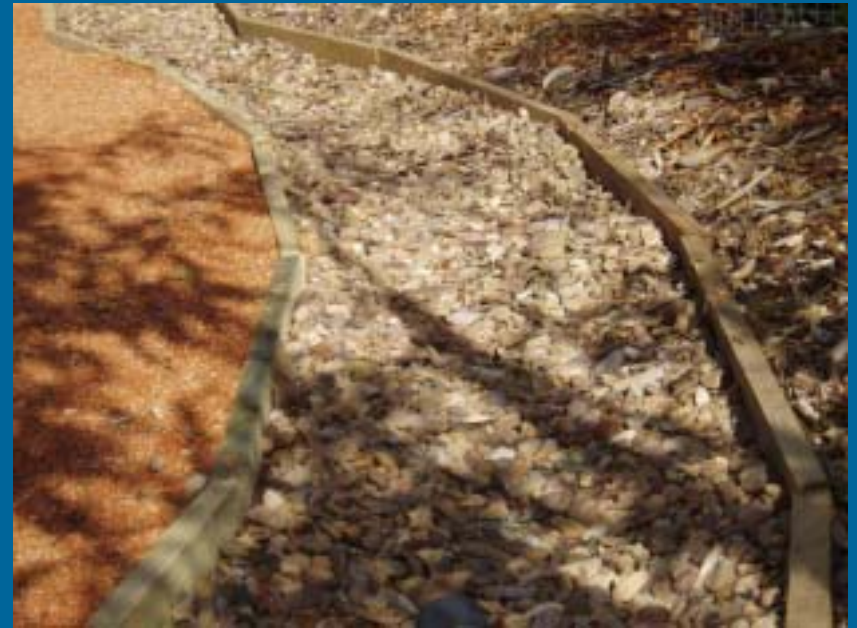
Gravel lined swales on our block. Timber edges installed to limit mulch input by Blackbirds
