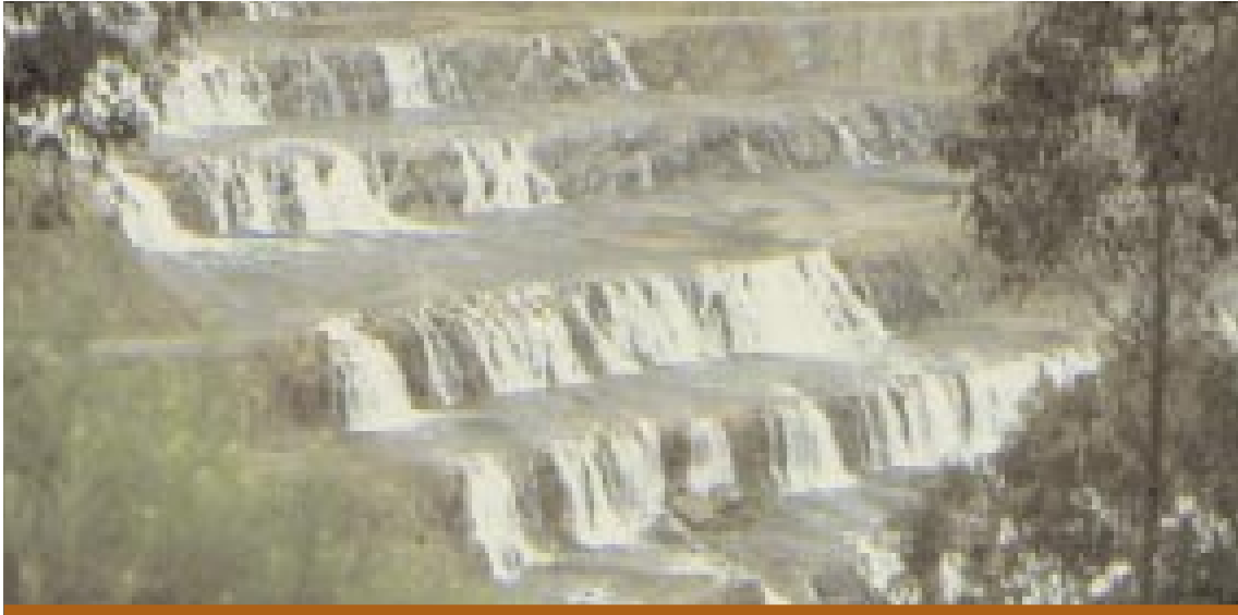
Dartmouth Dam spillway. Barriers to migration have been cited among the major problems facing the sustainability of Australia's freshwater fisheries resources. Photo: John Hawking
