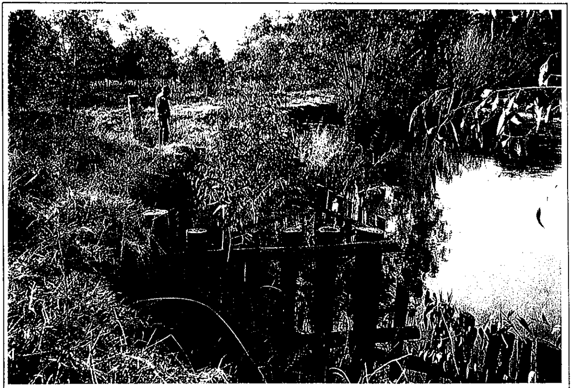
Plate 3. Groynes to aid establishment on actively eroding bank. Mungabareena Reserve, River Murray. (a) November 1992, (b) July 1995.
