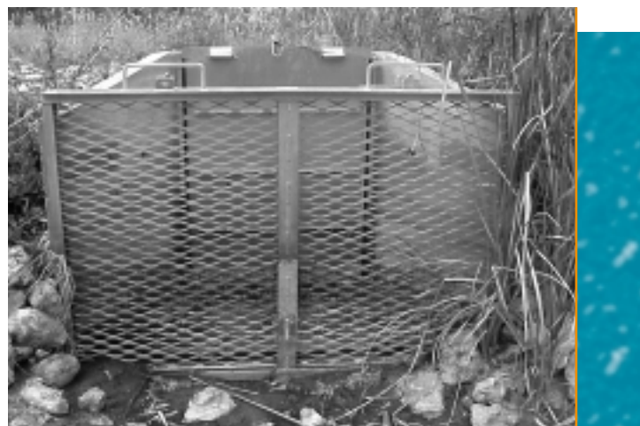
Carp exclusion screen at Causeway Lagoon, near Renmark, SA. Photo: Kane Scott.
