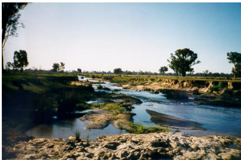
Fig. 4.8. Branjee Creek between Nelsons Rd and Drysdale Rd. This section of Branjee Creek was originally a narrow drain cut to divert all baseflows from Creightons Creek into Branjee Creek. The channel has deepened and widened substantially over the last 30 years.
