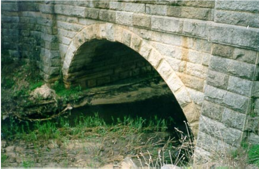
Fig. 4.12. Pranjip Creek at the Hume Freeway. More than 0.5 m of sediment may have been deposited in this section of channel between 1958 and 1998.
