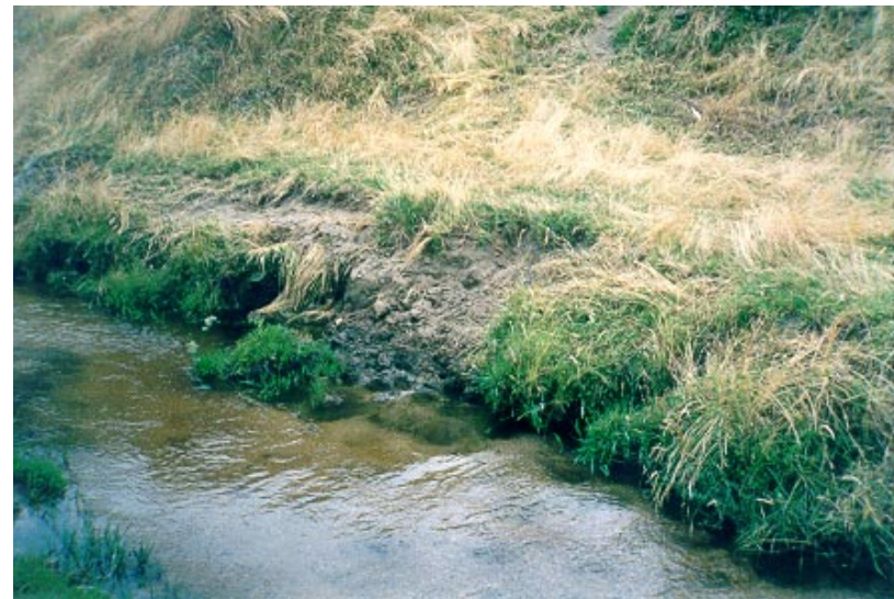
Fig. 5.7. Bank erosion on Creightons Creek due to stock trampling
