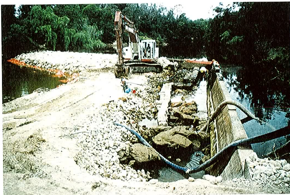
Photograph 5. The placement of rocks below the Lower Wyong Weir, Wyong River to prevent water leakage through the existing concrete structure.
