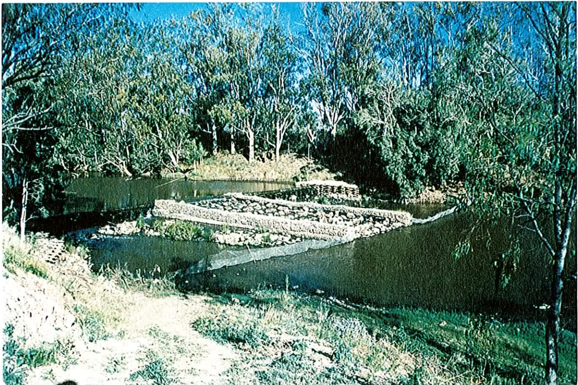
Photograph 12. Goondiwindi Weir and Fishway during sampling on 7 November 1995 with flows less than 300 ML/day. (Note lack of flow over side crests)
