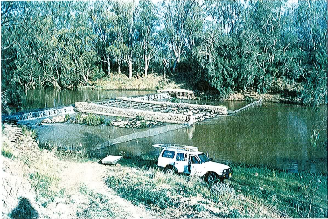
Photograph 11. Goondiwindi Weir and Fishway during sampling on 4 November 1995 with flows greater than 600 ML/day. (Note flow over side crests)
