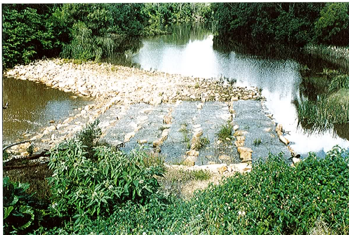
Photograph 6. In September 1993 extra rock was placed below the Lower Wyong Weir and a rock-ramp fishway formed. (Note the lower weir crest in the foreground)
