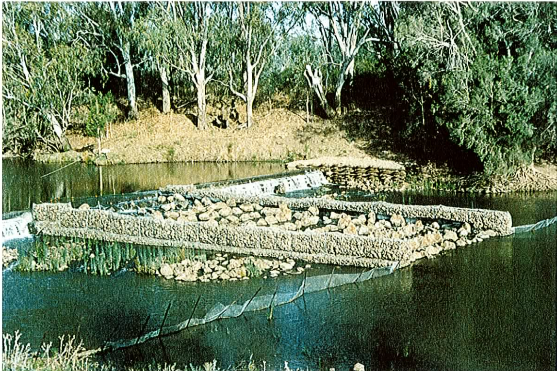
Photograph 10. The rock-ramp down the centre of the river with crests on each side of the channel raised to direct water through the fishway. (Note the guiding fence)
