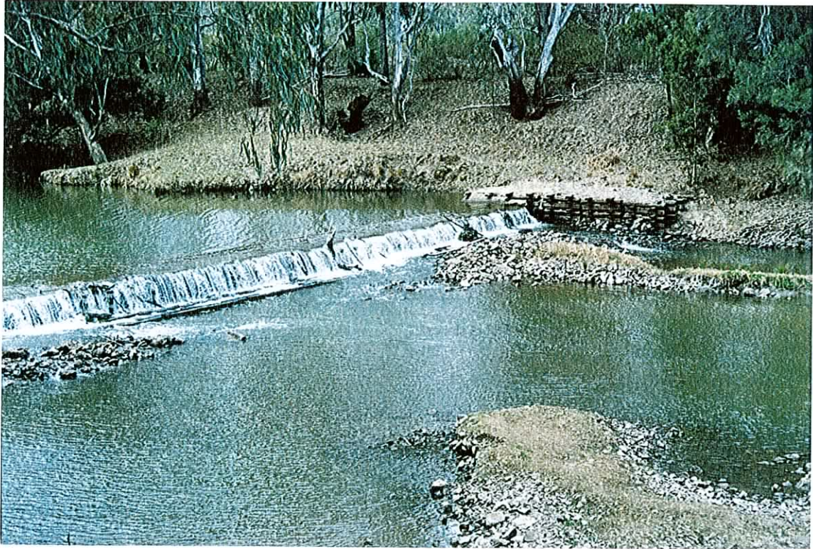
Photograph 9. The original wood-and-concrete weir at Goondiwindi on the Macintyre River before the construction of a rock-ramp in August 1993.
